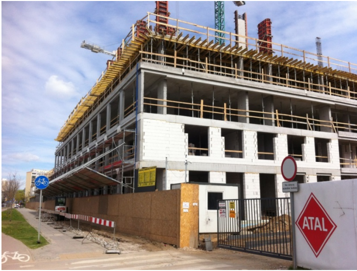
Atal's construction site in Warsaw. ©LeidenAsiaCentre
